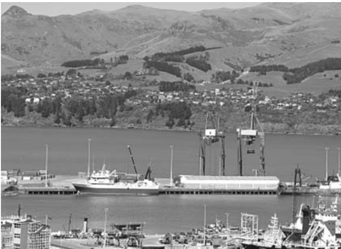
Figure 5: Residential development in Lyttleton Harbour
